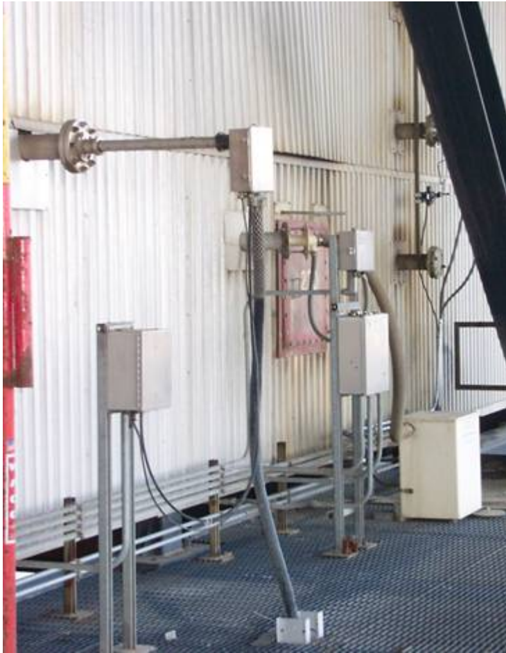
CEMS Probes In Outlet Duct
