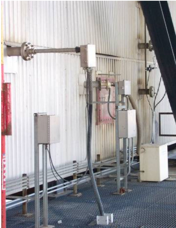
CEMS Probes In Outlet Duct
