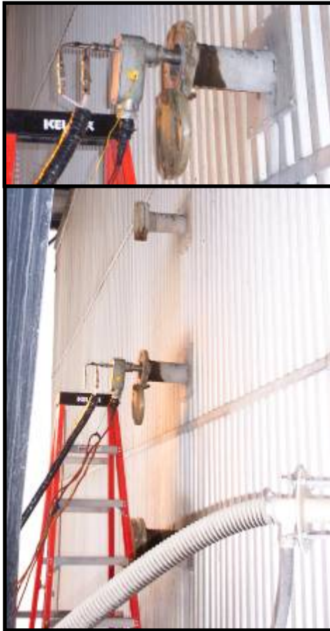
Emissions Probe In Outlet Duct
